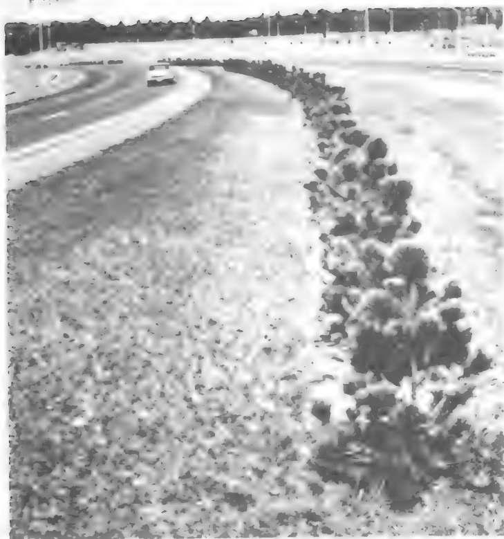
Evergreen trees planted on a curve provide a screen for headlights and safety for night driving; they serve as a beauty spot in daytime.
